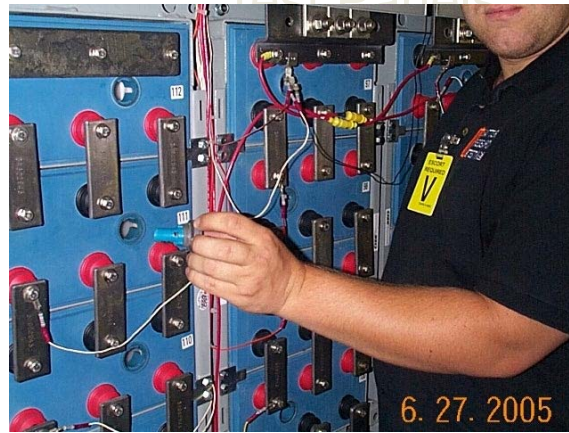
Catalyst Cap installation
