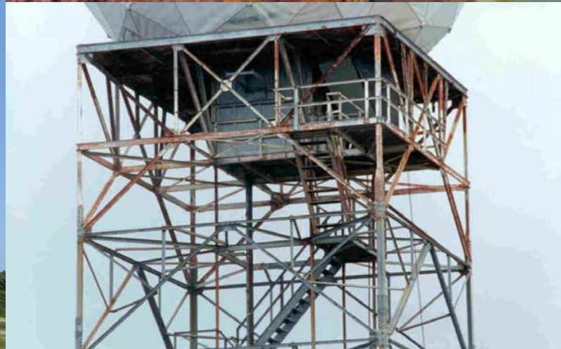
Current tower corrosion
