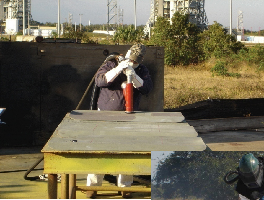
Depaint with Blast Recovery System (BRS)
