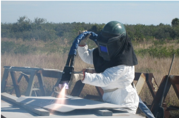
Application of Thermal Spray Coating to Heat Shield
