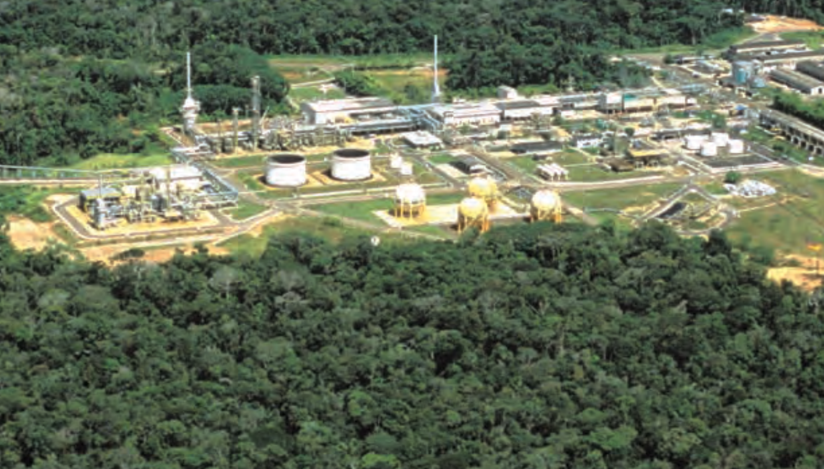
Urucu Operational Center.
