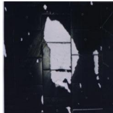
Large Impact Gouge – Downstream of missing tile
