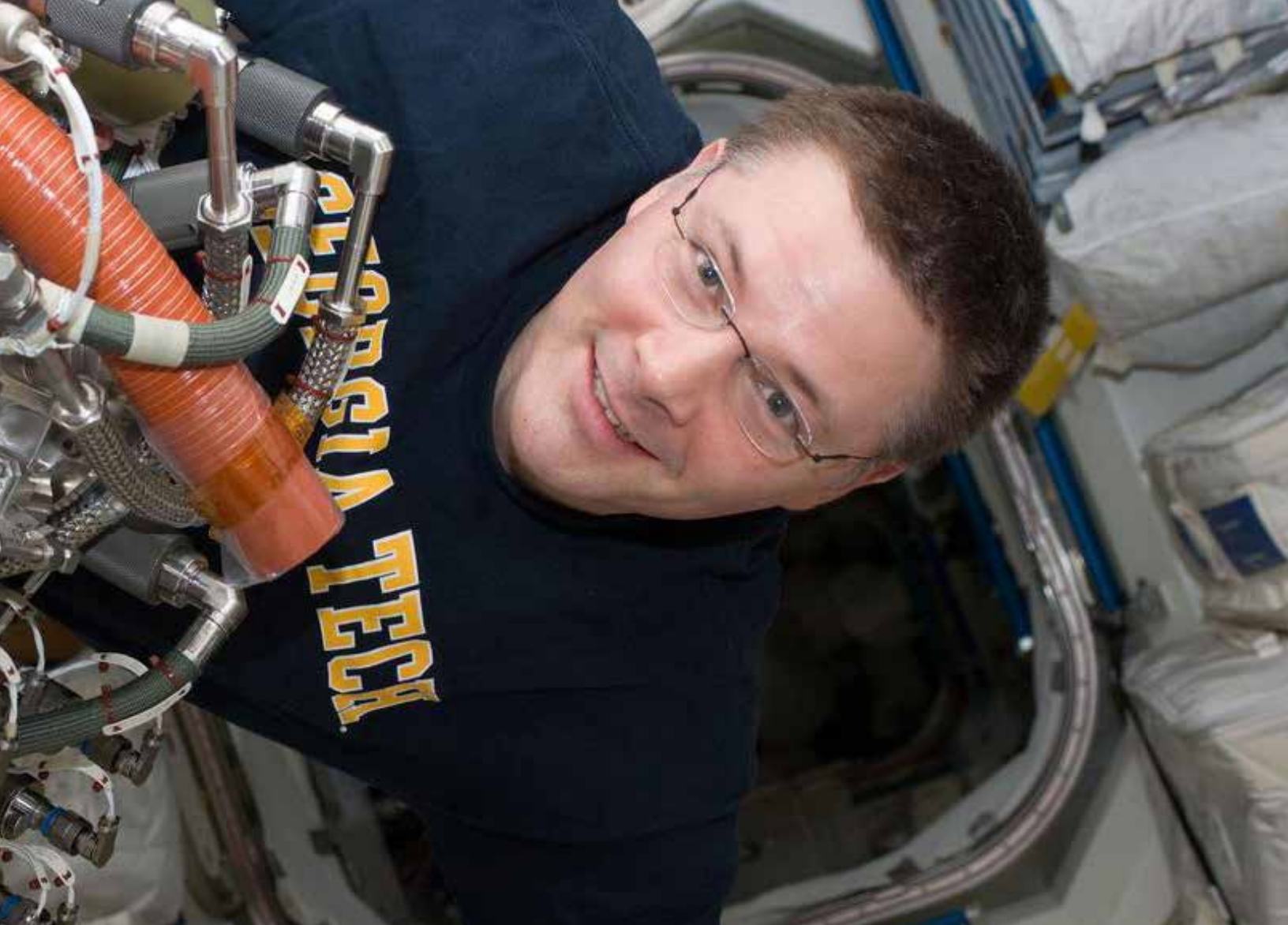
NASA Astronaut and Expedition 25 Commander Doug Wheelock works to install a system to extract more water out of the International Space Station atmosphere as part of the station's Environmental Control and Life Support System.
