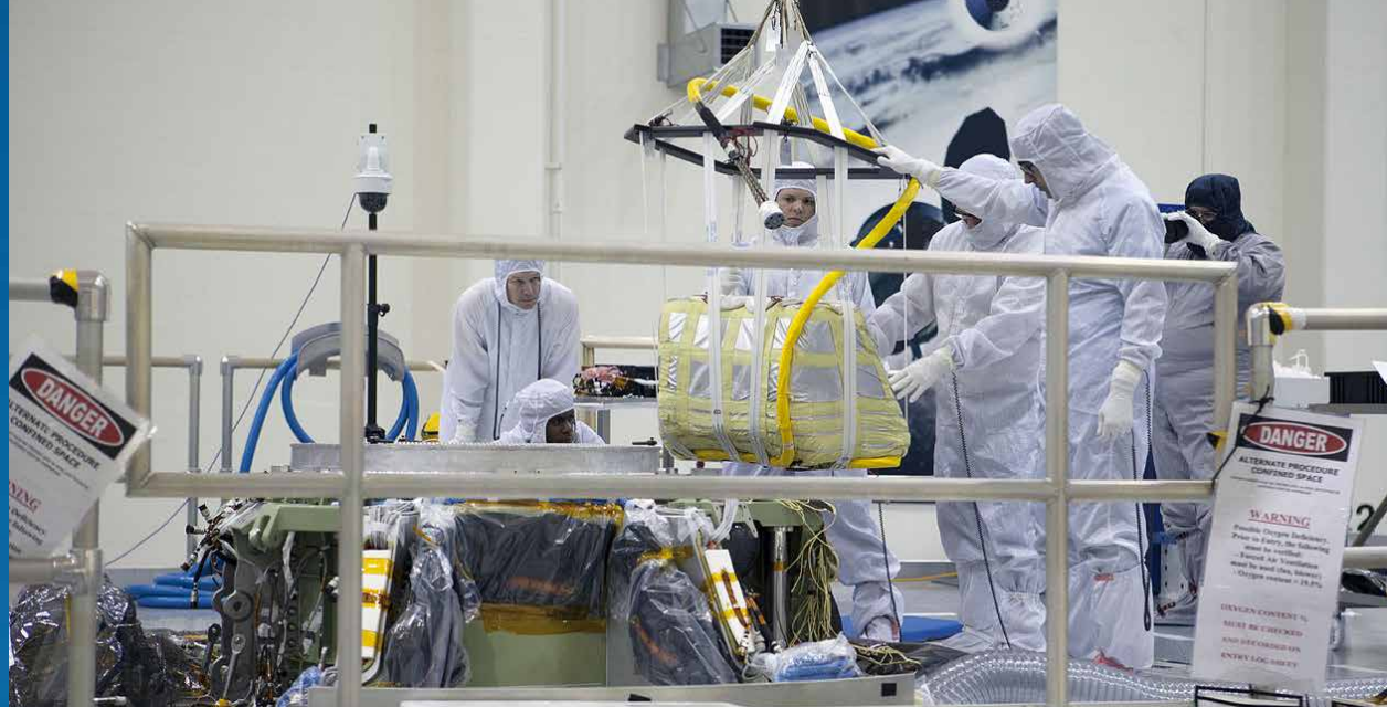
A crane lowers a main parachute for installation on the Orion spacecraft inside the Operations and Checkout Building high bay at NASA's Kennedy Space Center in Florida.
